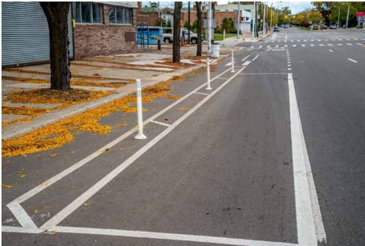
Painted buffer with flexposts and parking lane (Jefferson Avenue, Detroit) Photo by MDOT Staff
