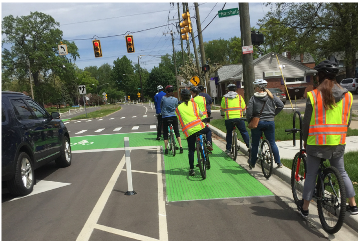
Painted buffer with flexposts and bike box (Livernois Street, Ferndale) Photo by MDOT Staff
