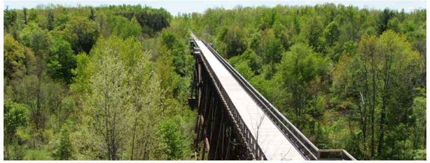
Mill Creek Trestle, Avoca Courtesy of St. Clair County Parks and Recreation
