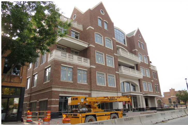
Above - Downtown Lofts under construction
