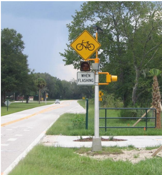
Fig. 5.7G. Active Crosswalk Warning Systems
