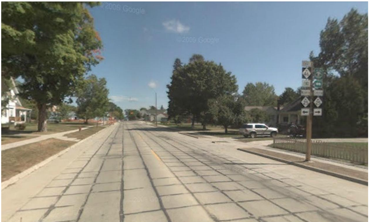
Looking east on Main Street (M-46) in the Downtown
